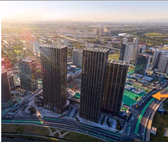
Day view of project
